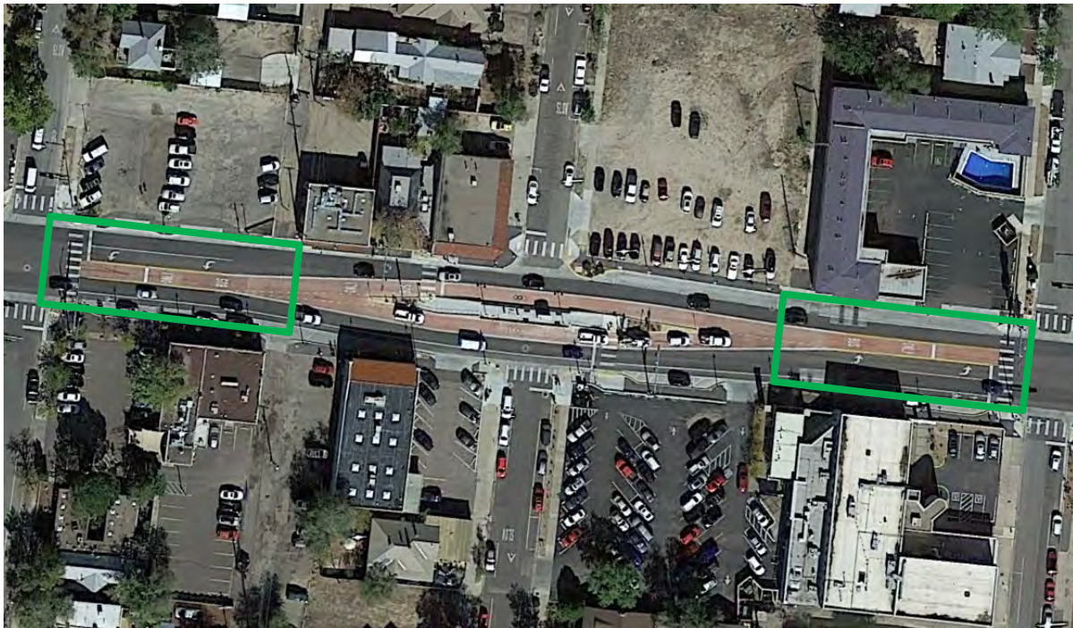
Figure B.9 Bi-directional BRT Lanes near ART Stop, Albuquerque, New Mexico Source: Google Earth
